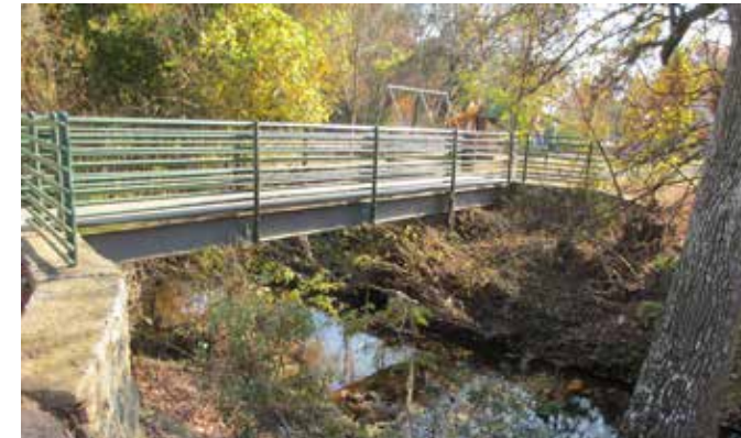
(3) Pedestrian bridge over the McDaniel Branch
